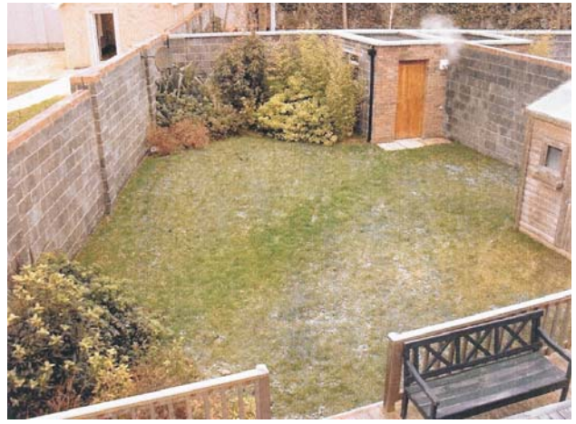
Line of heating pipe visible via melted snow
