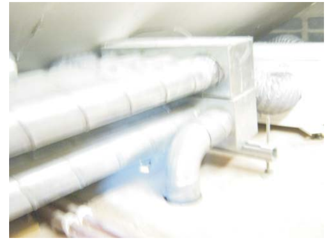
DORMER ATTIC SPACE ABOVE BATHROOMS
