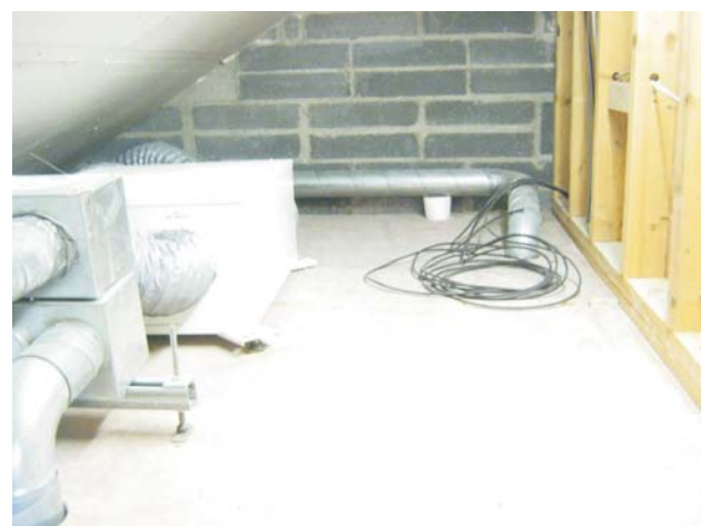
DORMER ATTIC SPACE ABOVE BATHROOMS
