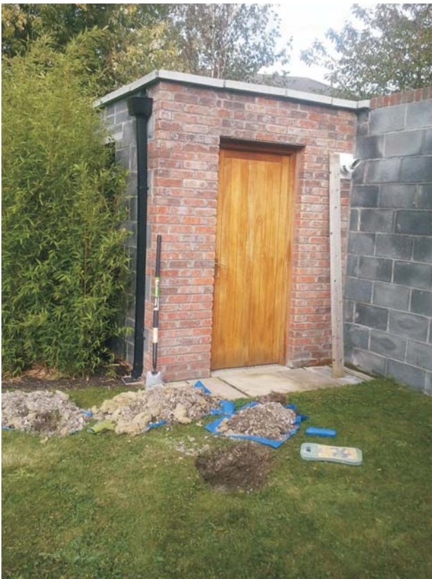
Hole dug adjacent to boiler house
