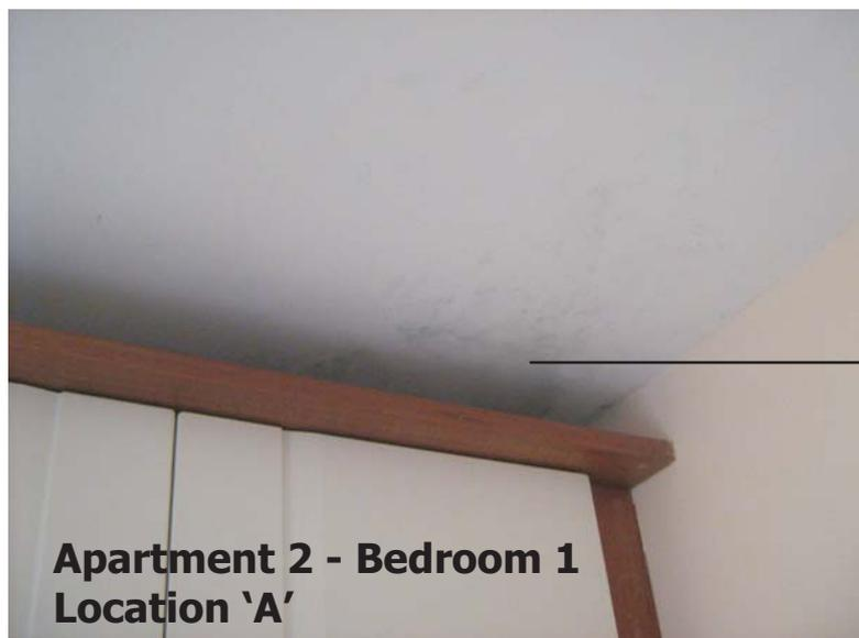
Mould spores clearly visible above fitted wardrobes
