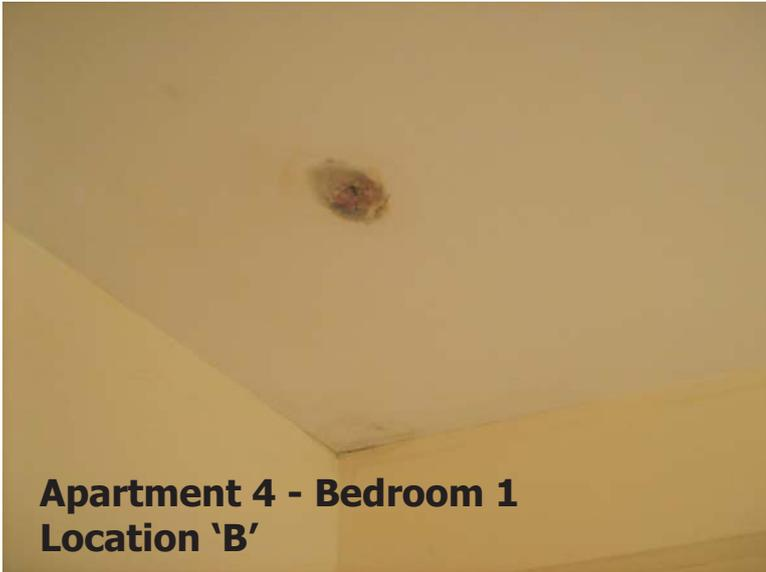
Hole in ceiling from damp penetration
