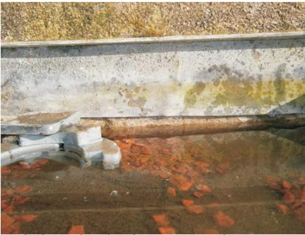
Flashing detail at location G with concrete paving removed
