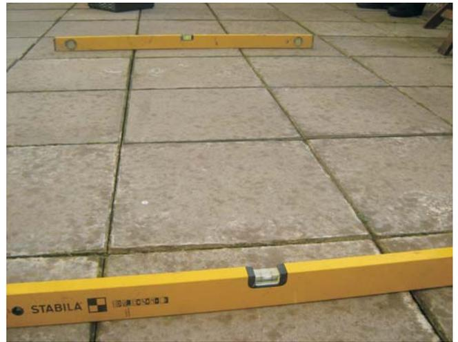
On examining the flat roof to the balconies to apart nos. 1 & 3 respectively, we noted that the construction appeared to be concrete roof tiles fitted on top of a heavy duty waterproof membrane.
