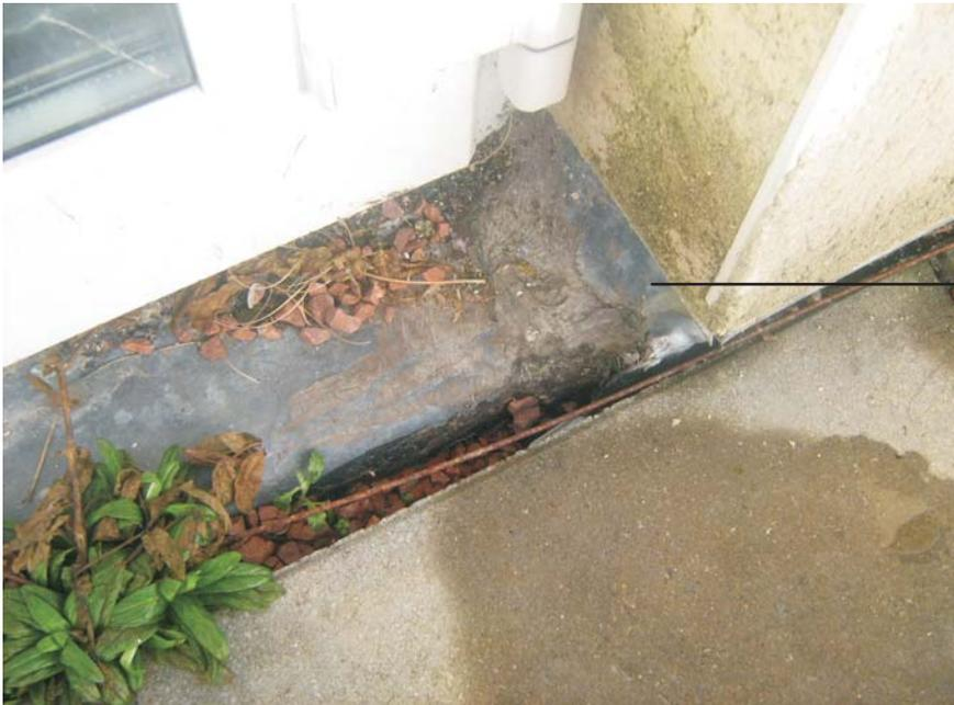
Flashing pinched at door jamb at location H.
