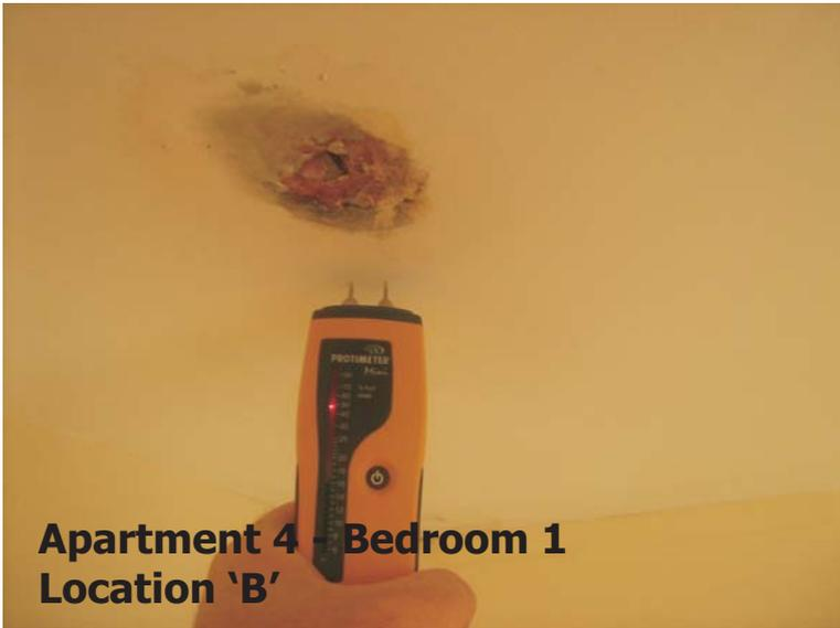
Moisture meter reading 50% moisture at location 'B'
