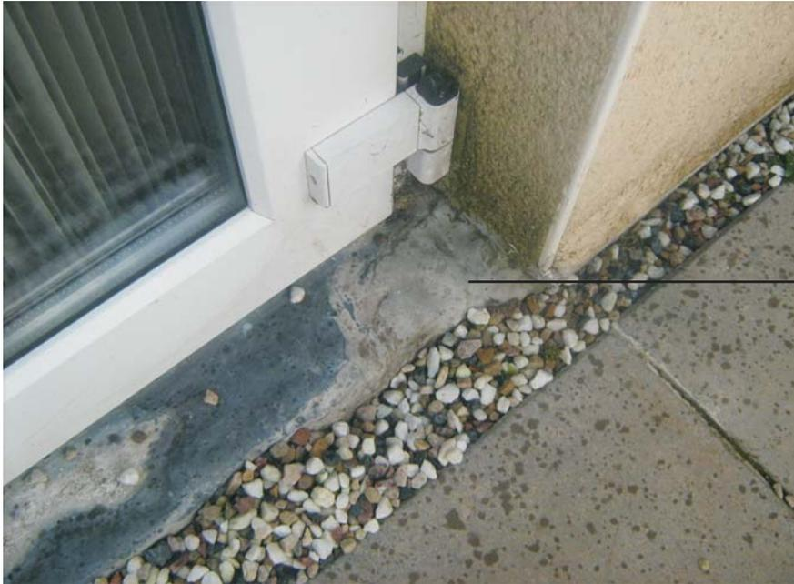
Flashing damaged and repaired with flexible sealant at location J.
