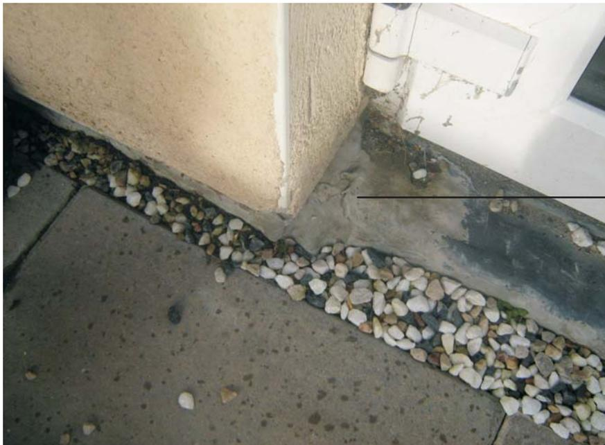
Flashing damaged and repaired with flexible sealant at location K.
