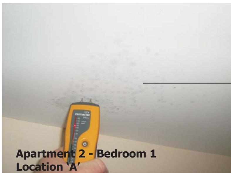
Moisture meter reading 50% moisture at location 'A'
