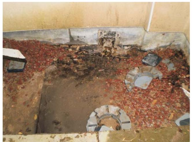
Location of balcony drain with concrete paving removed - wall structure inhibiting flow of water to hopperhead
