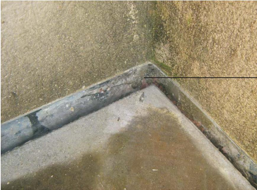
Flashing completely disintegrated at location G.
