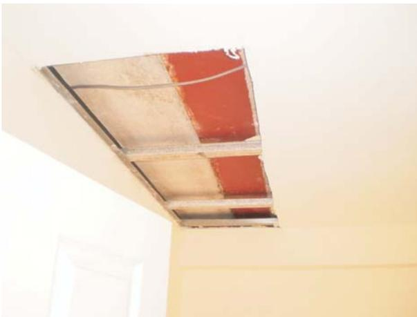
Portion of ceiling removed to show water damage along steel beam
