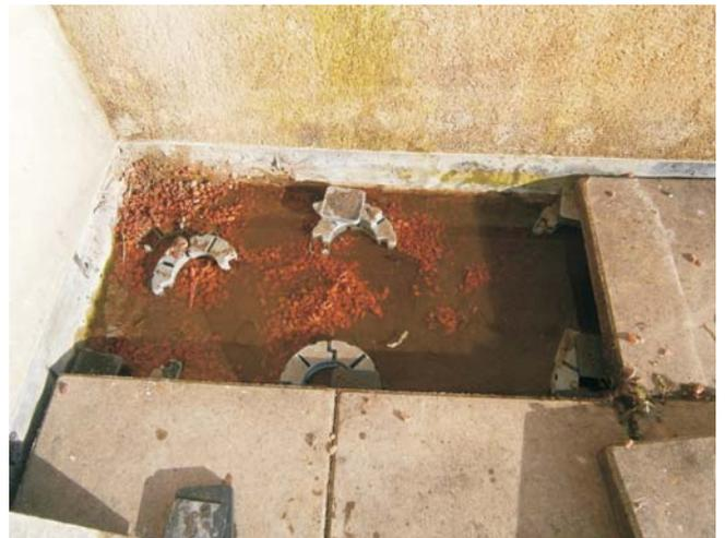
Flashing detail at location G with concrete paving removed
