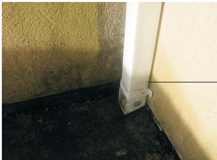
Rainwater pipe (indicated on dwg-page 2) discharging water onto balcony from adjacent roof and ponding at location.
