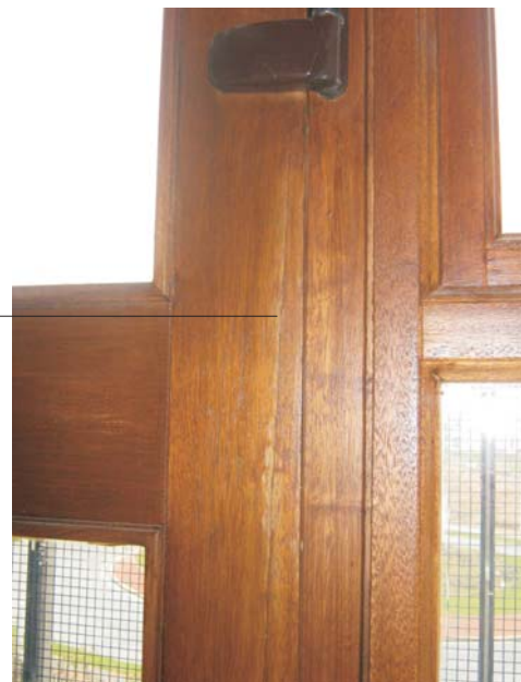
Crack to RHS of doorset
