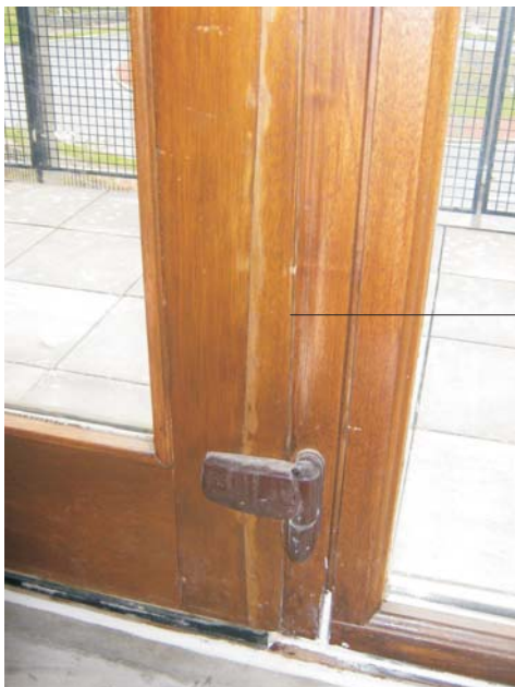
Crack to RHS of doorset
