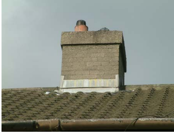
Chimney stack with flashing in reasonable condition.
