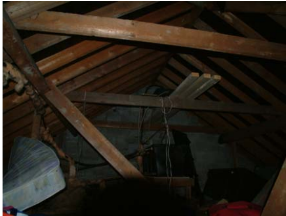
Attic photograph with header tank at top of photograph, connected cold water tank centre, and un-connected cold water tank to right hand side.
