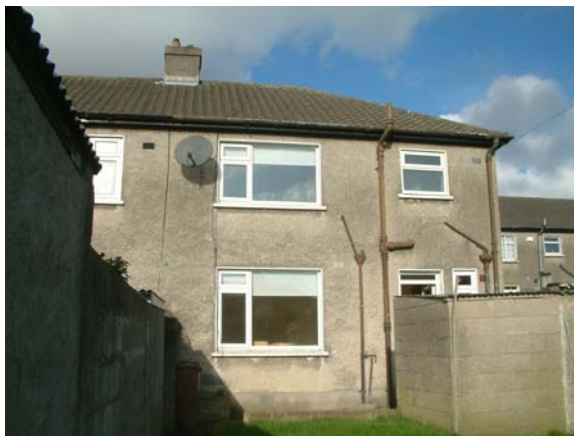
Pitched hip-ended roof with concrete roof tiles in reasonable condition.
