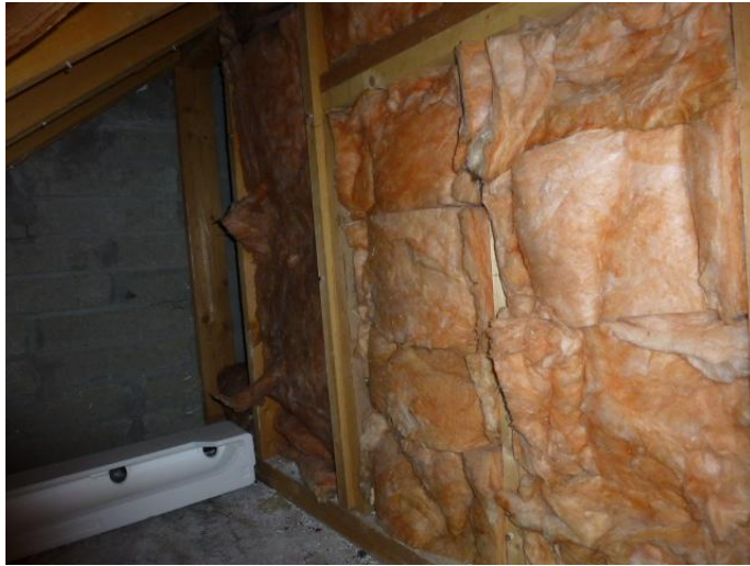
Attic photograph – insulation evident
