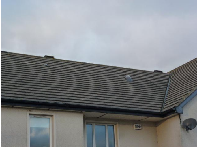
Roof fabric in reasonable condition
