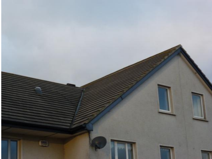
Front elevation – vent tile/flashings in reasonable condition
