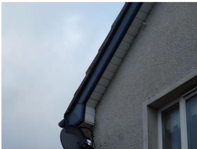
uPVC fascias and soffits in reasonable condition
