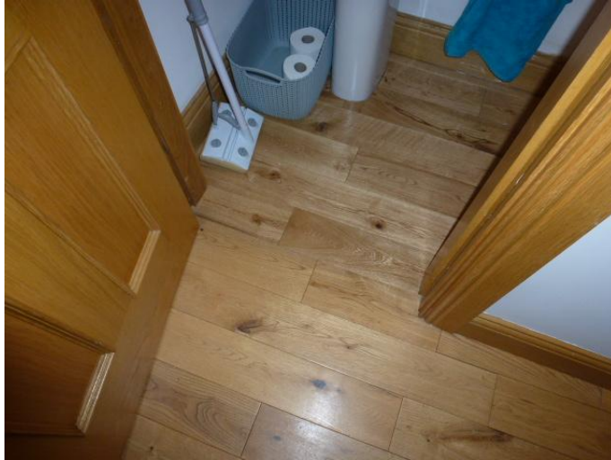
Floor finishes in reasonable condition
