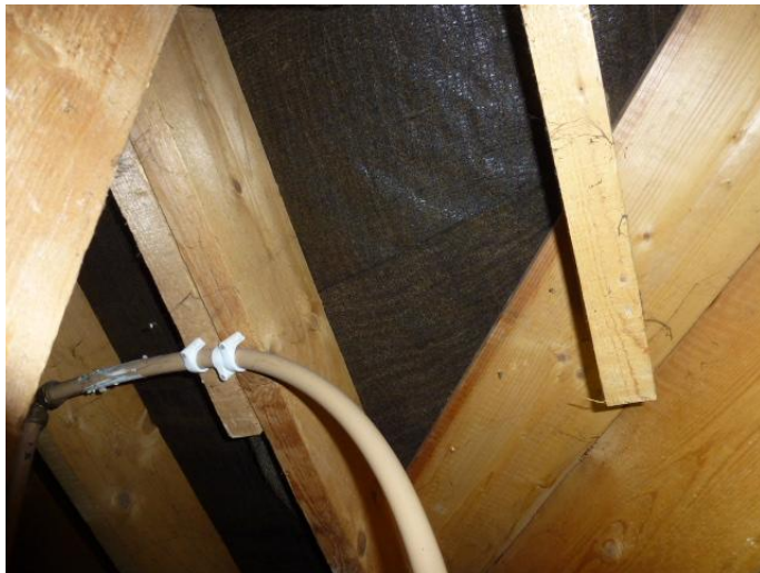
Attic photograph – sarking felt beneath rafters
