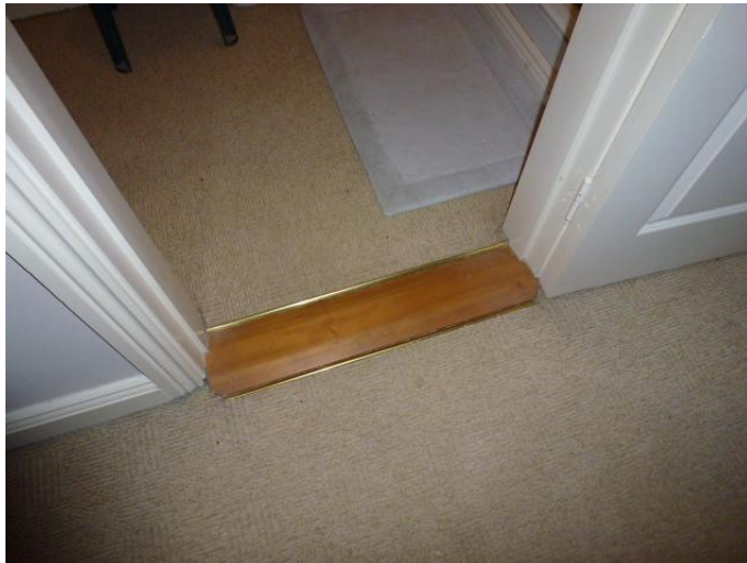
Floor finishes in reasonable condition
