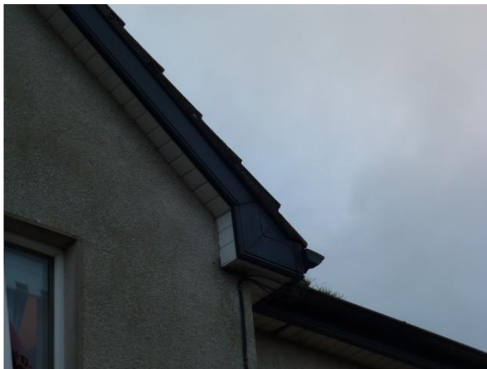
Rain water/soil goods in reasonable condition
