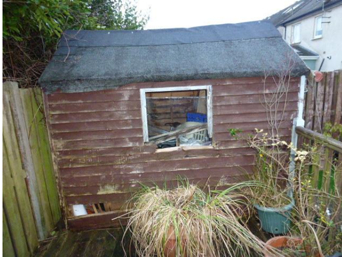
Timber shed in reasonable condition.
