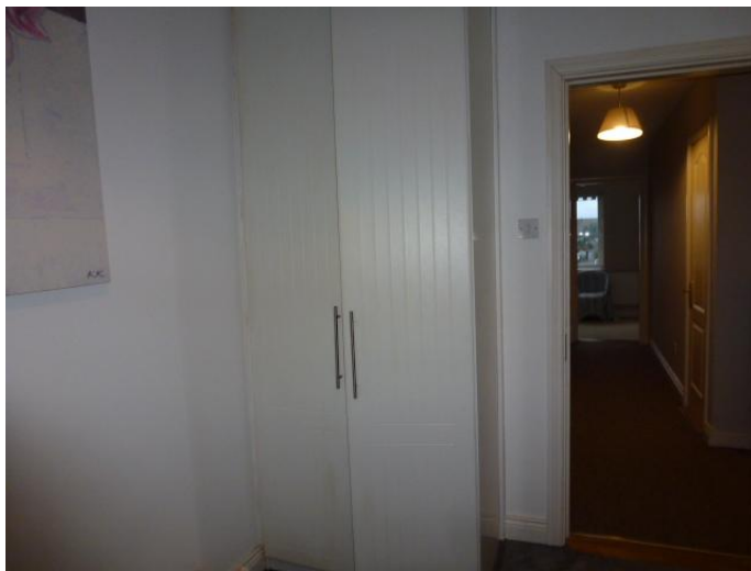
Bedroom units in reasonable condition
