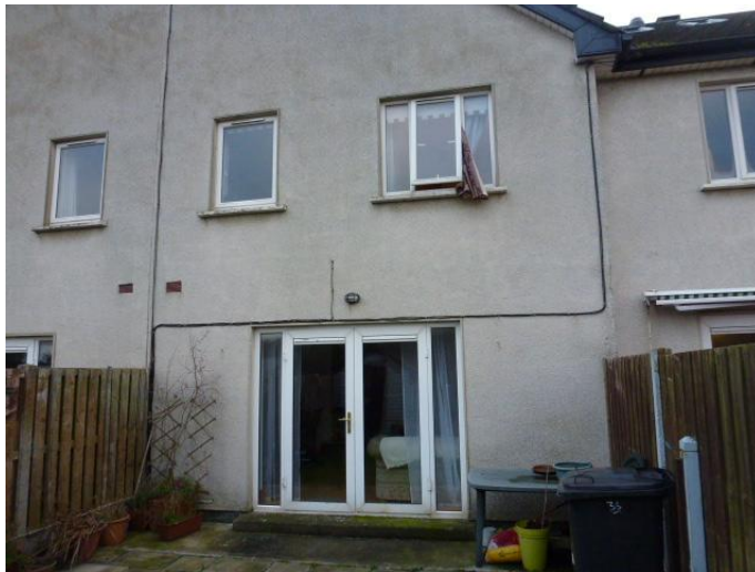
Render finish to rear elevation in reasonable condition
