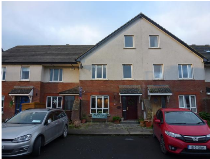
Brick/render finish to front elevation in reasonable condition
