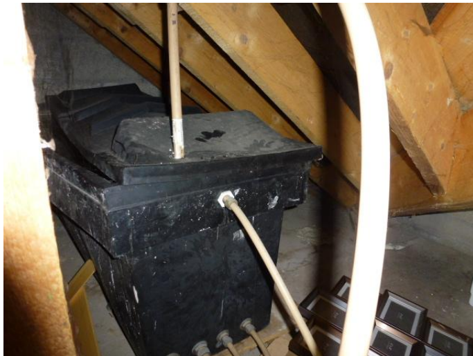
Attic photograph – cold water tank
