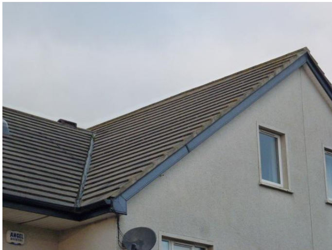
uPVC fascias and soffits in reasonable condition
