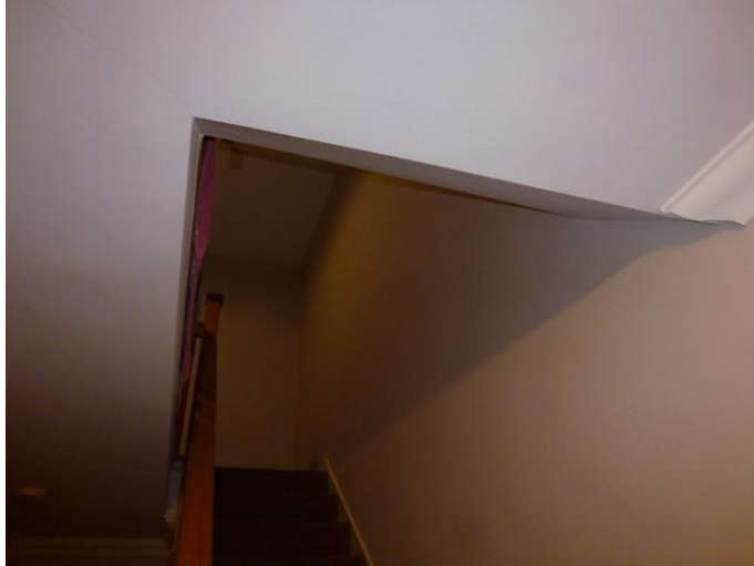
Plaster finishes in reasonable condition
