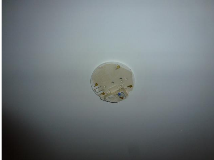
Fire detector – living room - removed
