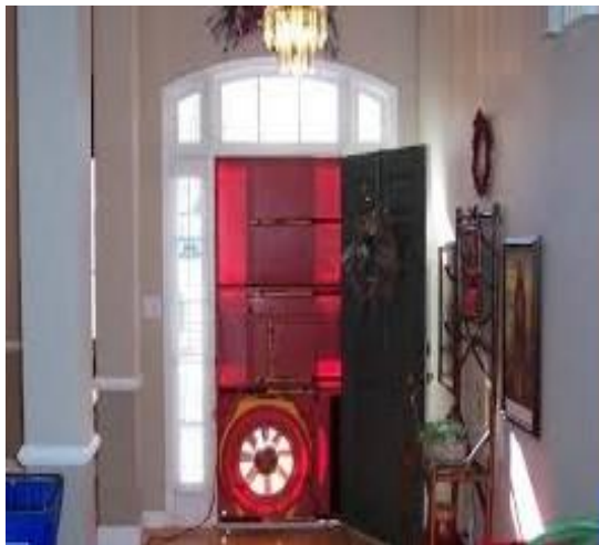
Typical blower door installed in hall door open
